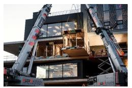
Figure 11: To reduce the impact of refurbishmentanddeconstruction,theUrbanMiningandRecycling(UMAR)ExperimentalUnitusesprefabricated elementsmade of recycled materials.(Architects: Werner Sobek, Dirk E. Hebel & FelixHeisel, Photo: Wojciech Zawarski)
